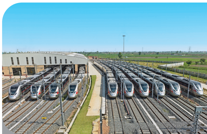
Delhi-Ghaziabad-Meerut Regional Rapid Transit System Project, India
