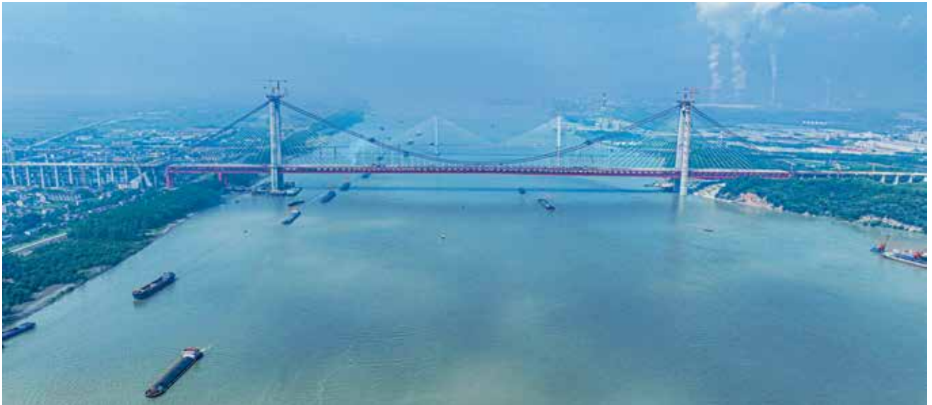
ANHUI TONGLING G3 ROAD-RAIL BRIDGE PROJECT IN CHINA
