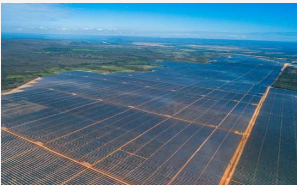
Picture of Pirapora Solar Complex in Minas Gerais State, funded under NDB's BNDES Renewable Energy Projects
