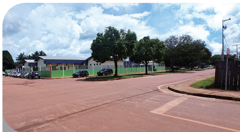
Paved street in front of school. The asphalt brought more safety, comfort and well-being to the school's students. – Rurópolis, Pará, Brazil
