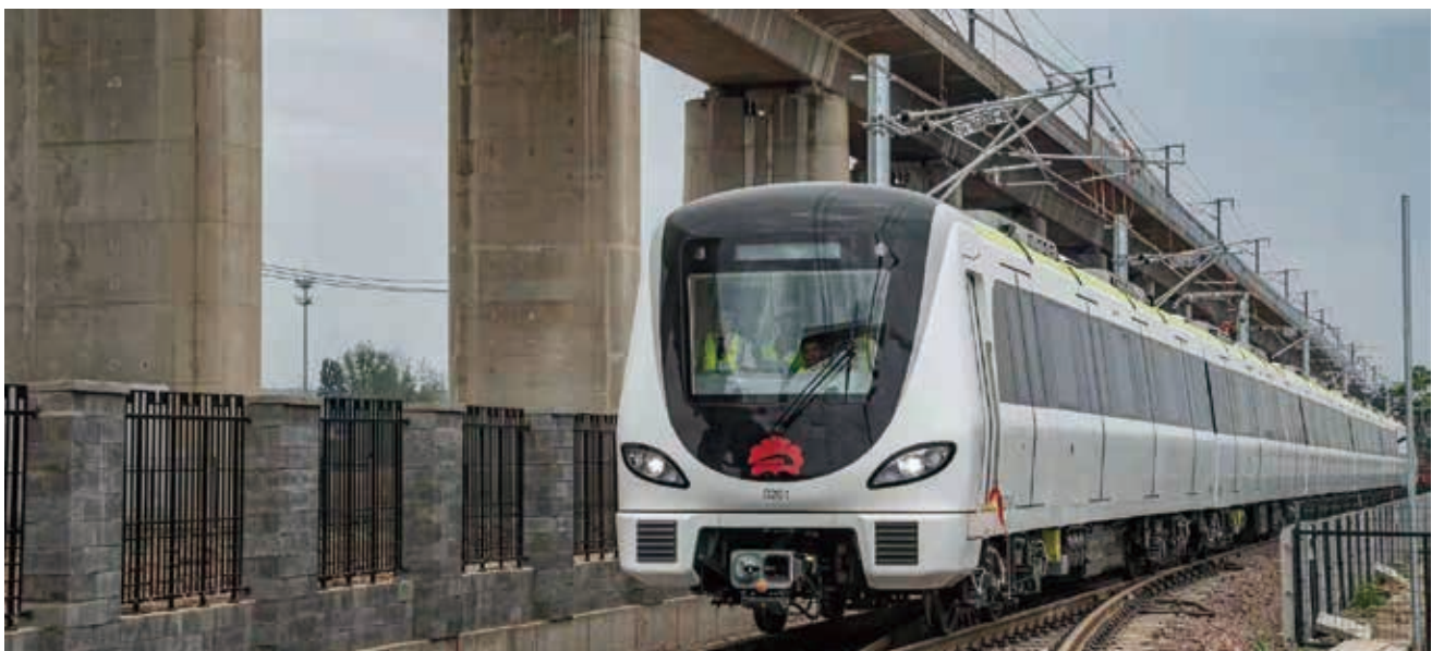
LUOYANG METRO RAIL, CHINA
